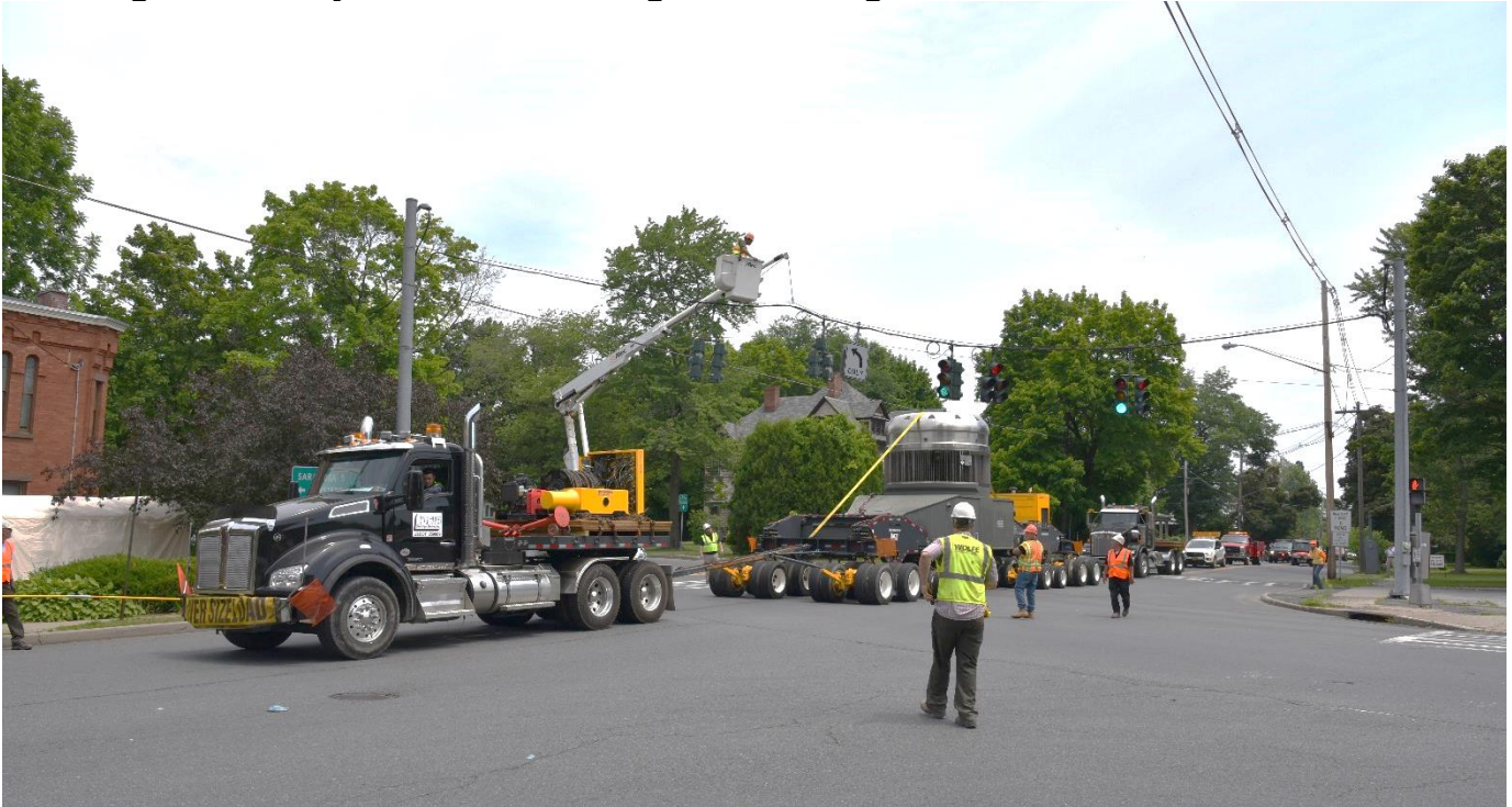
Figure 3: Heavy Haul Tractor Pulling Trailer through Intersection of Routes 50 and 67
